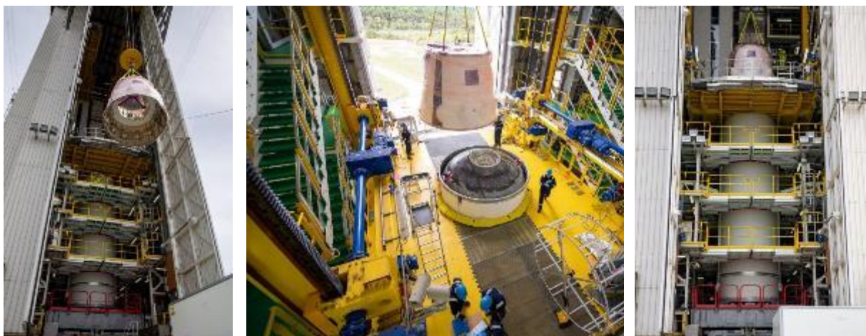
Figure 6.2.3.2.1.b – Hoisting and integration of the 1/2 interstage
